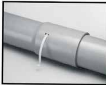
Slide locking ring into the joint.
